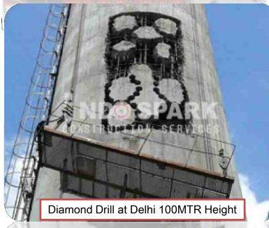
Diamond Drilling is the most versatile and efficient method of forming holes and opening in a wide range of hard material From heavy reinforced concrete and natural Stone and Bricks.
